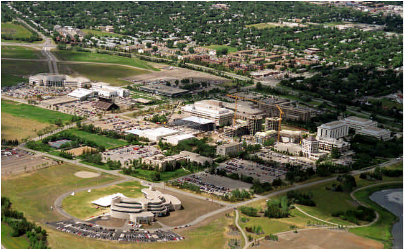
34. The Main Campus and Research Park Looking South West - 2003
