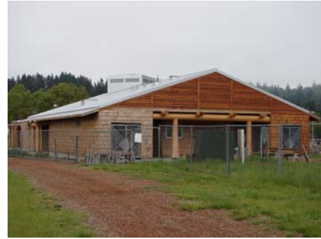
Figure B.8.2: Native American Longhouse (under construction)
